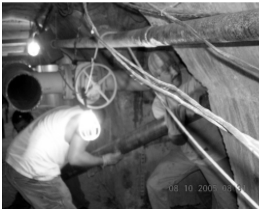
Waldinger Tunnel Job at Kansas State University
