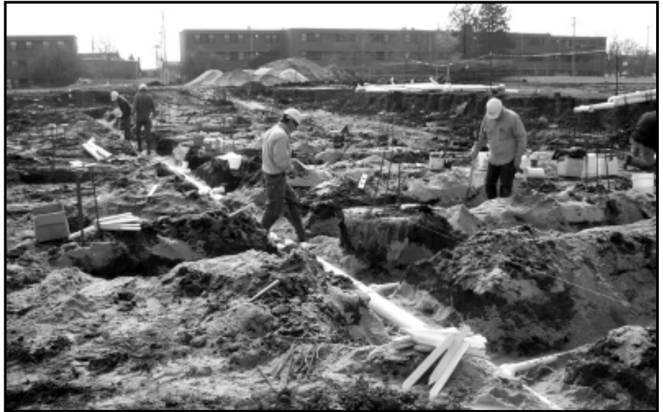
#441 Members Install Underground at Fort Riley
