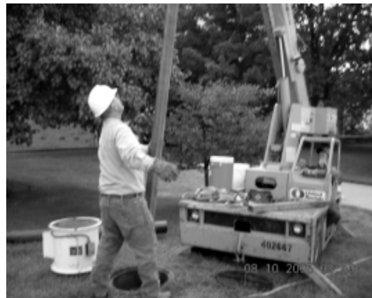
Moving Pipe for Waldinger at K-State
