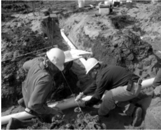
Members install underground at Fort Riley
